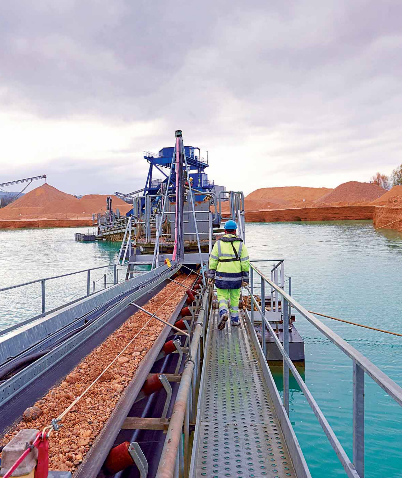
Aggregate mining in Saint-Jean-le-Vieux in Ain, France
