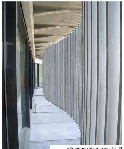
▲ The imposing 2,500-m² façade of the ITER administrative building at the Cadarache facility (France) consists of 2,000 high-performance concrete units in 100 different dimensions.
