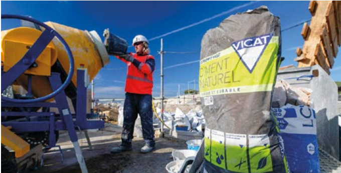
▲ Work in progress at Château d'If, Marseilles (France)
