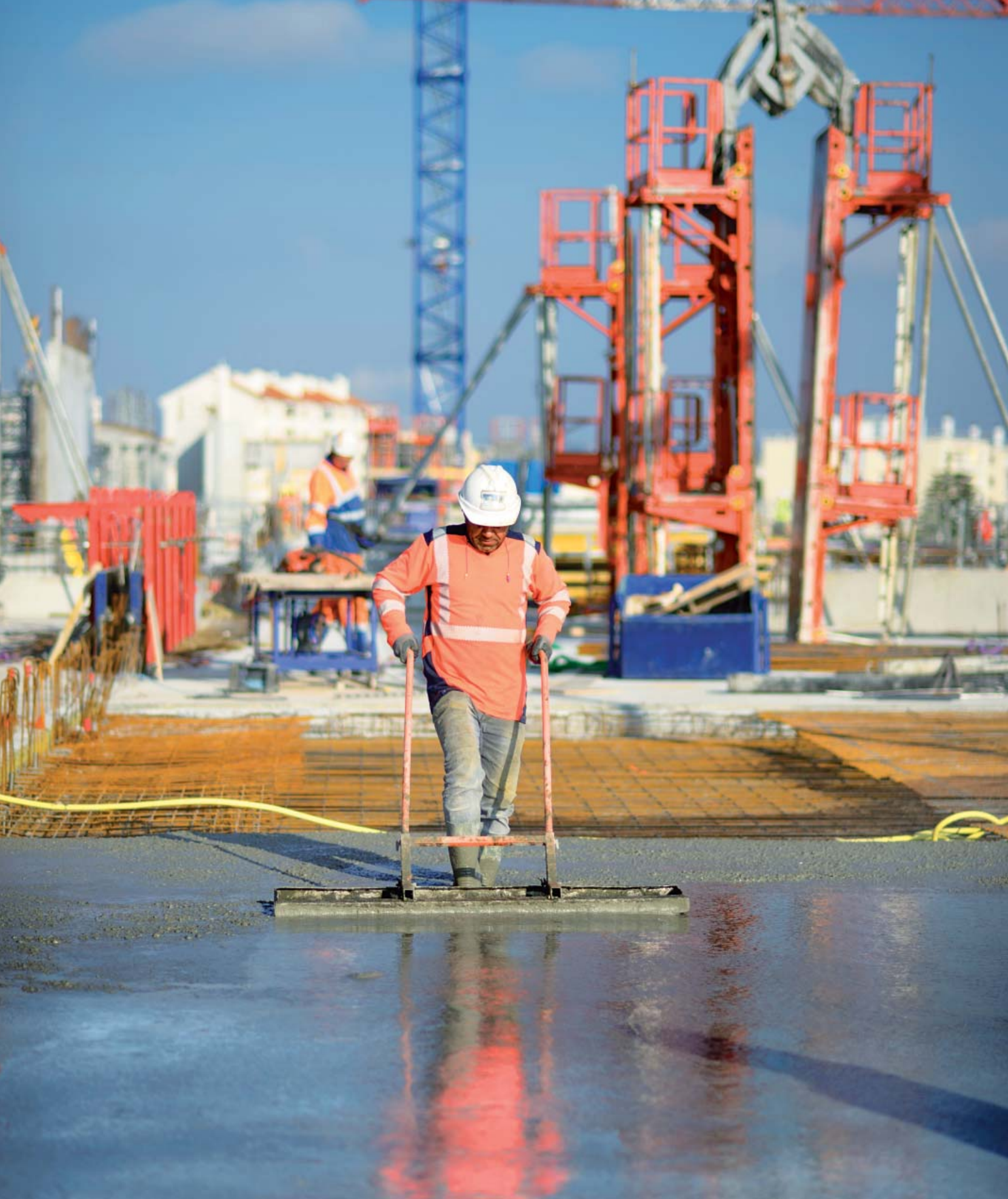
Finishing a concrete slab at the Medipôle site in Lyon, France
