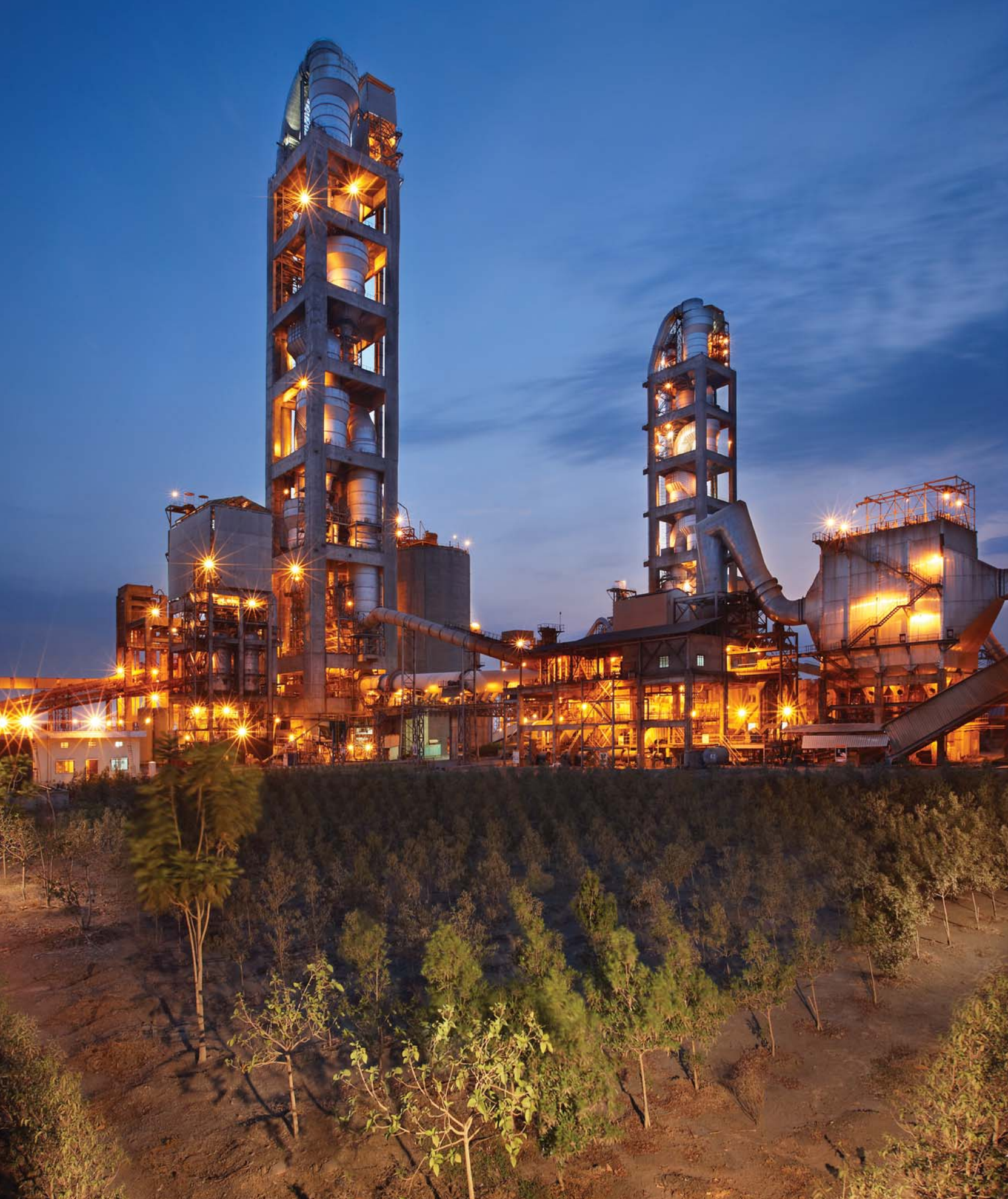
Bharathi Cement factory in the State of Andhra Pradesh, India
