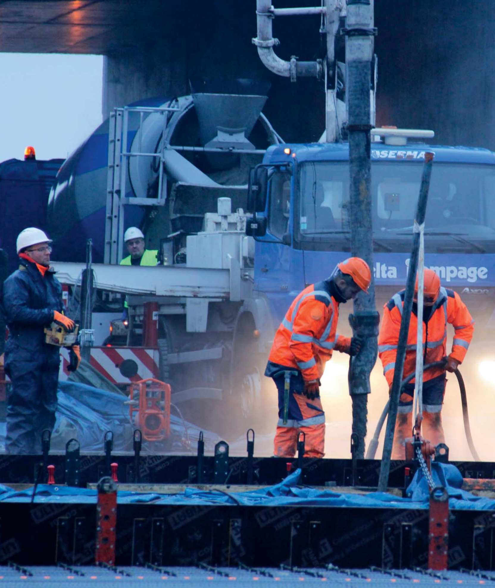
Use of ready-mixed concrete with Delta Pompage, France
