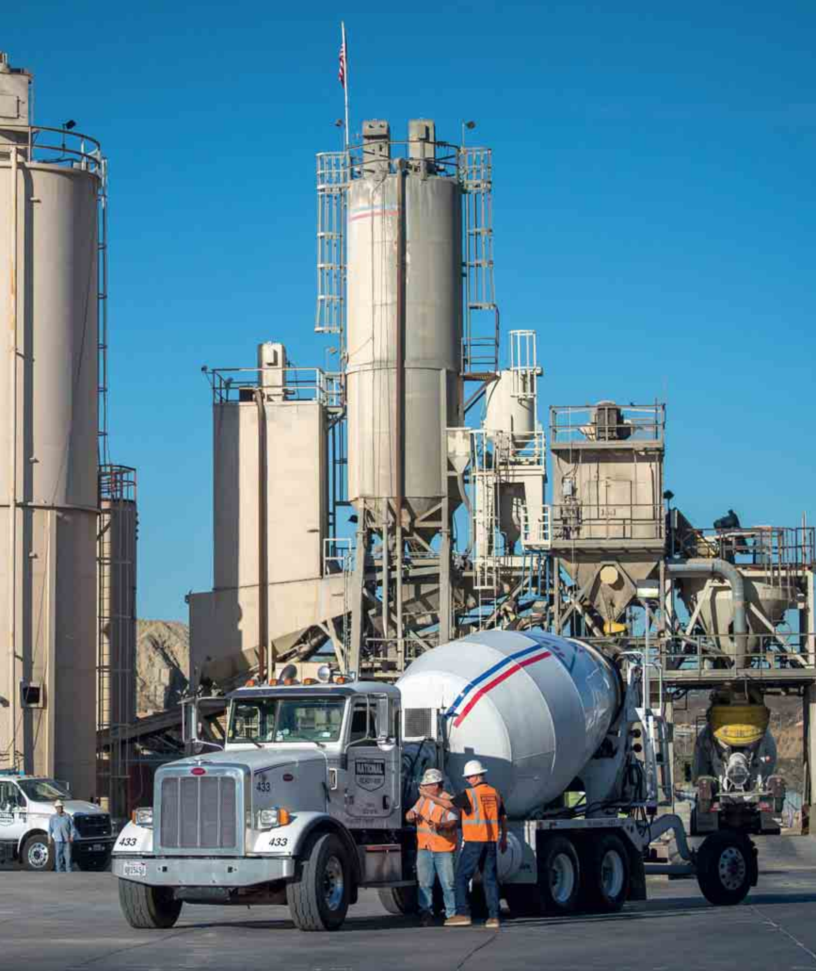
National Ready Mix concrete batching plant, Santa Clarita, California, USA
