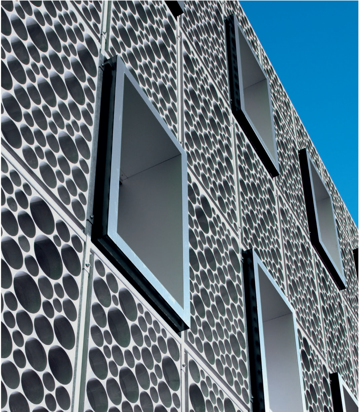
▲ The front of a Swatch group building in Cormondrèche (Switzerland), built using Ultra-High Performance Fibre Reinforced Concrete (UHPFRC), six times more resistant than common concrete.
