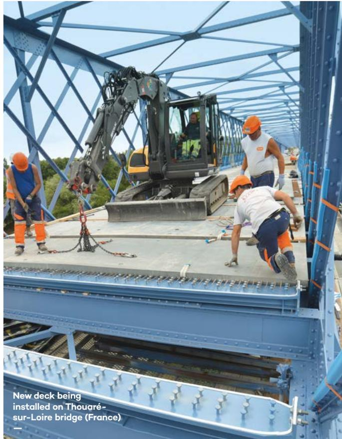
New deck being installed on Thouaré-sur-Loire bridge (France)
