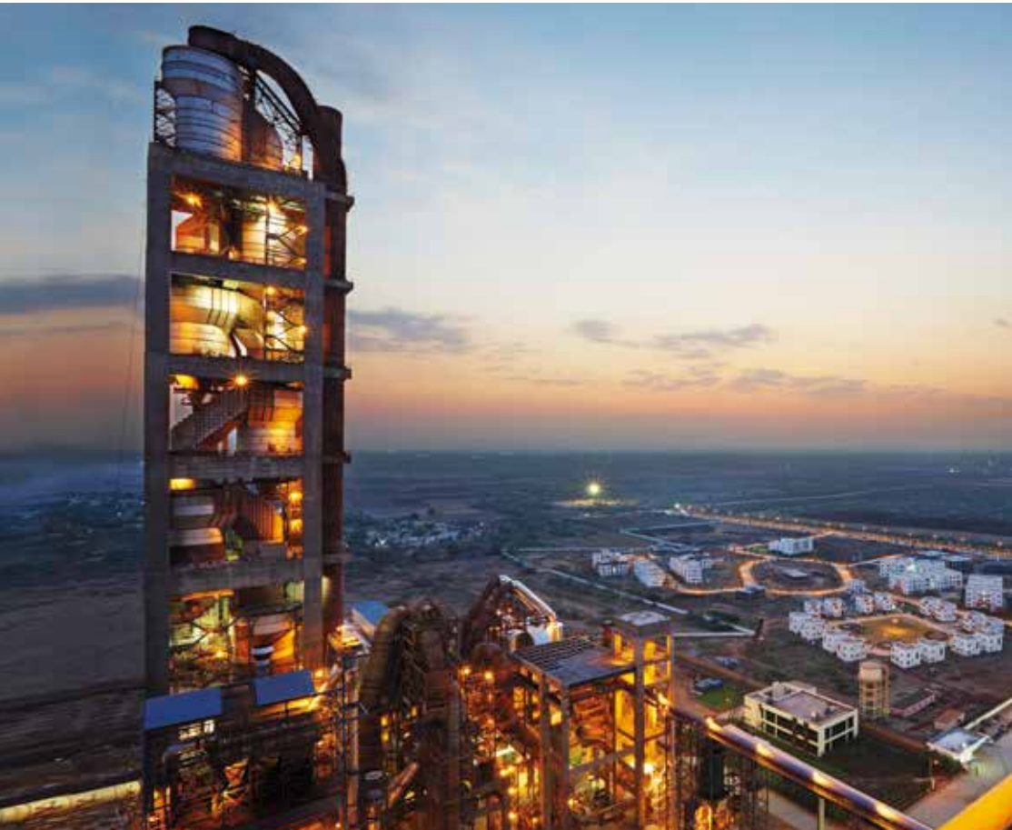
Bharathi Cement plant, Andhra Pradesh.
