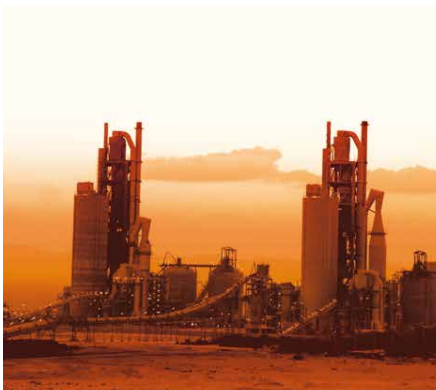
Sinai Cement Company plant near El Arish (Egypt).
