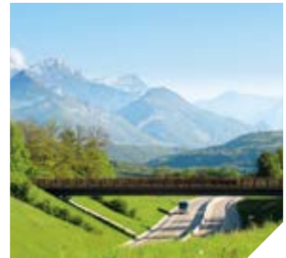
— Chabotte Bridge, Isère (France), built with SMART UP ultra-high-performance fiber-reinforced concrete.
