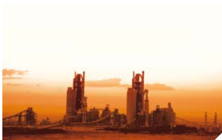
— Sinai Cement plant, near El Arish (Egypt).
