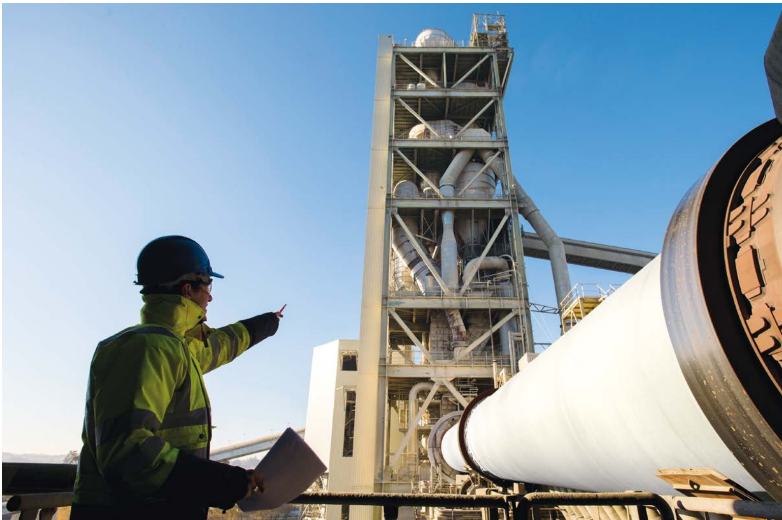
Kiln and preheater tower, Montalieu cement plant.
