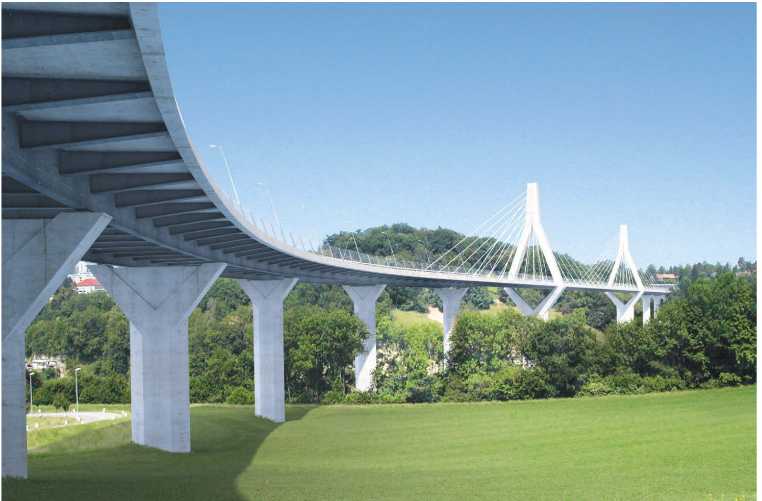
La Poya Bridge (Switzerland).
