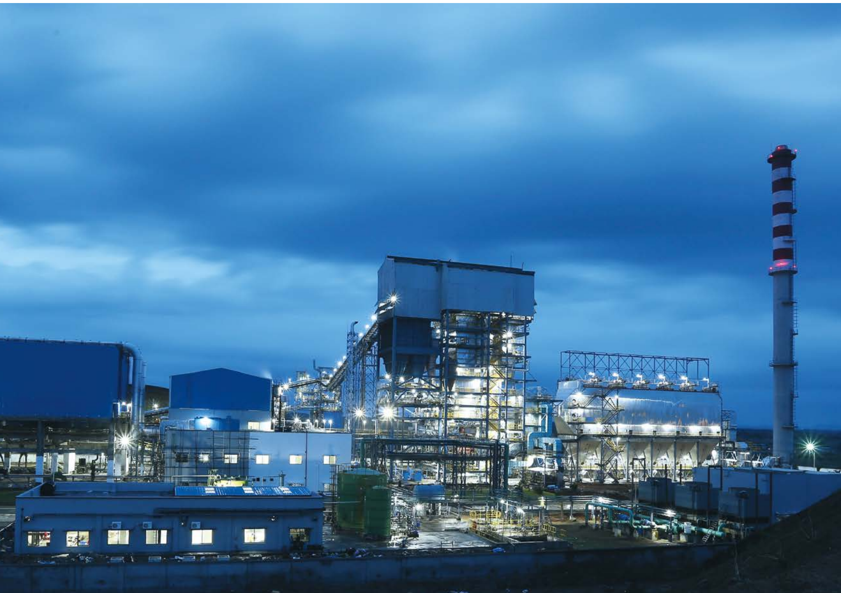
Bharathi Cement power plant.
