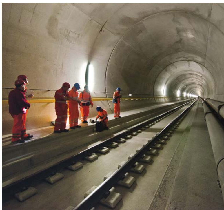
LVT ballastless railroad track in the Gotthard Base Tunnel.
