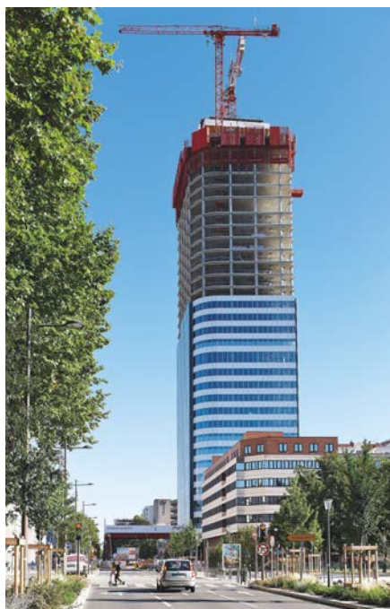
Work in progress at Incity Tower, in central Lyon.
