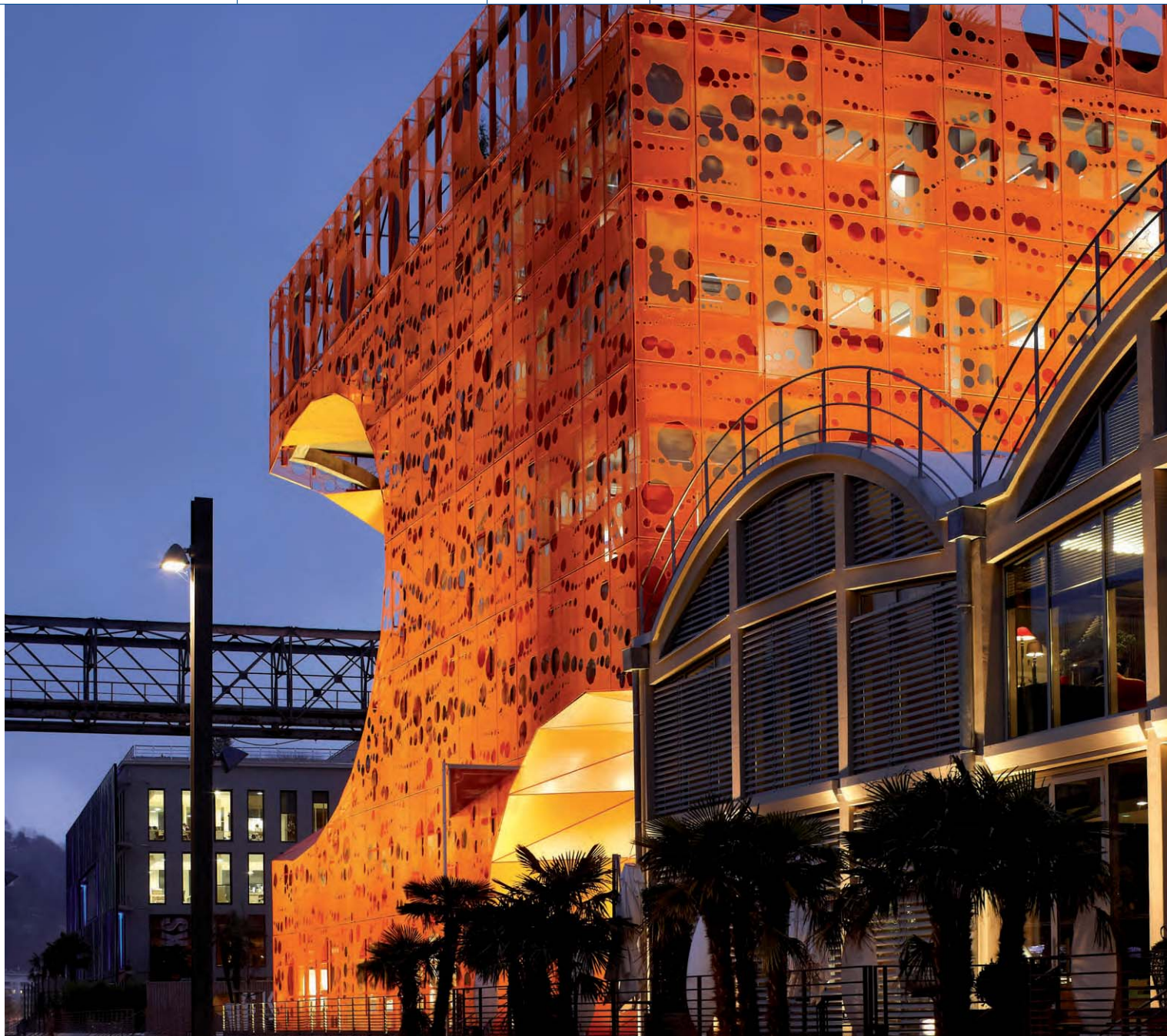
▲ "Cube Orange" building in the Confluence district of Lyon, France (architects Jakob + MacFarlane).
