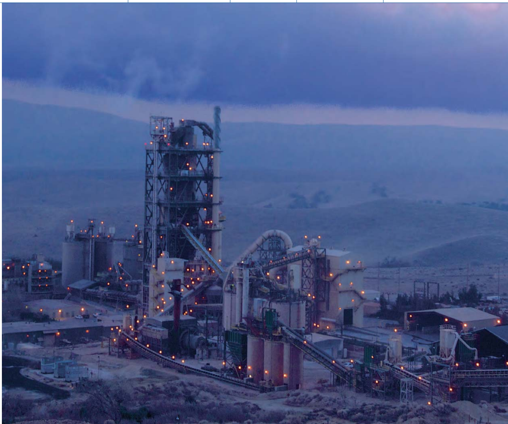
▲ Lebec cement plant, California.
