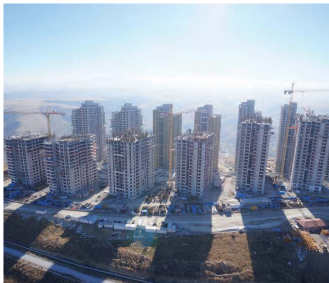
▲ Residential project under construction near Ankara.
