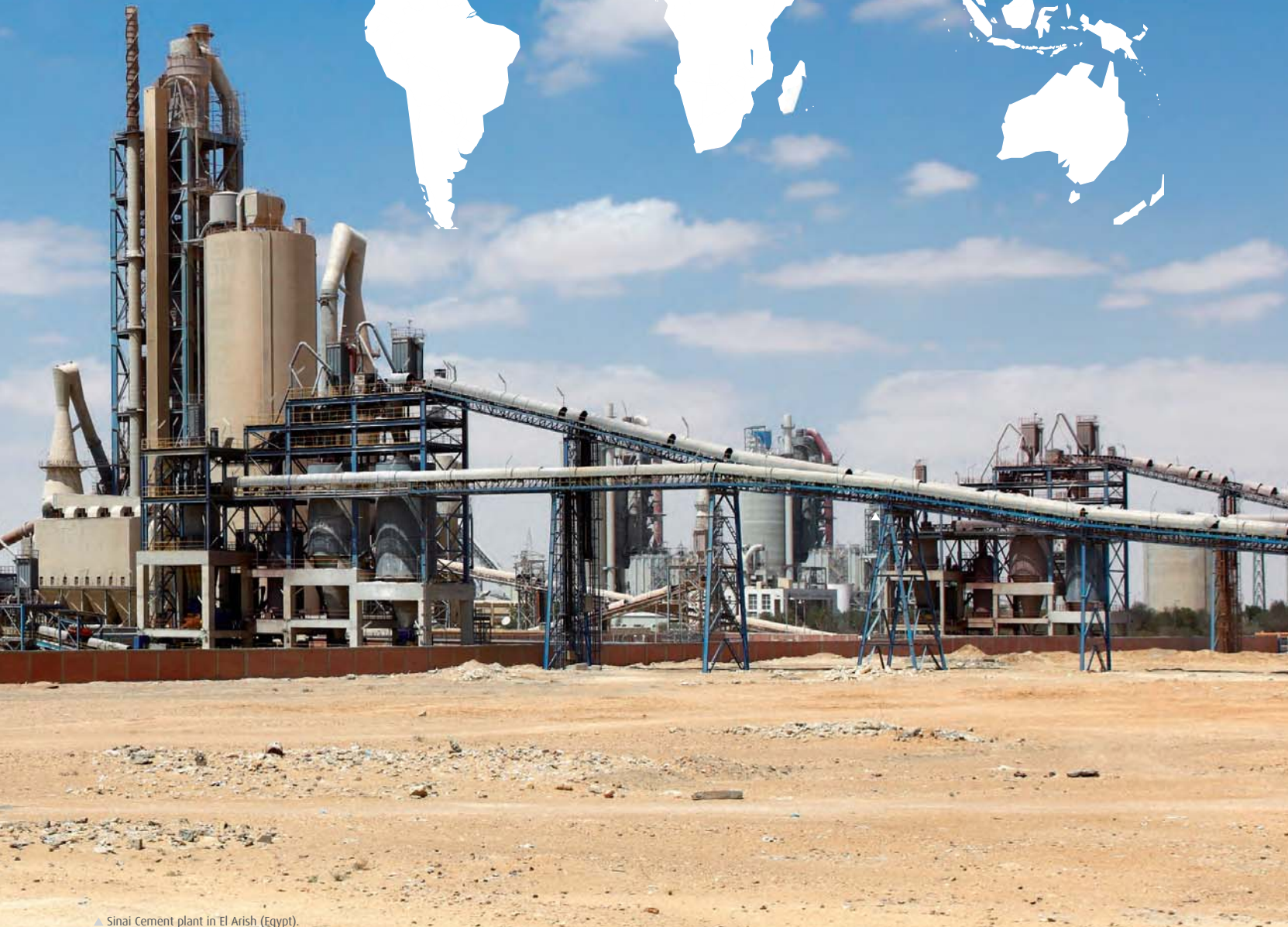
▲ Sinai Cement plant in El Arish (Egypt).
