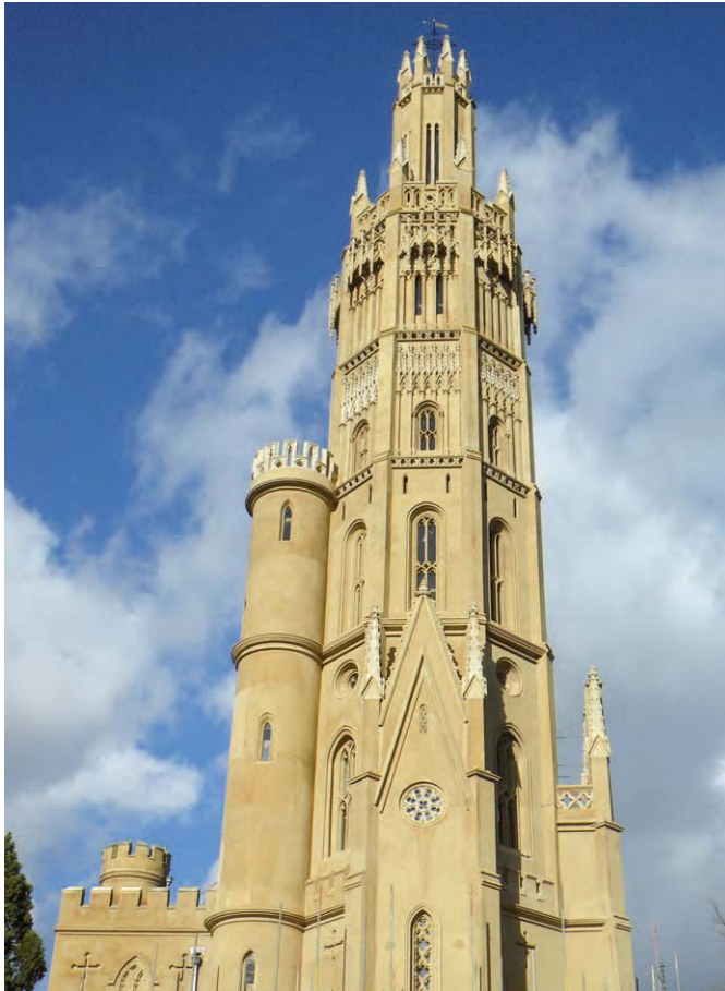
▲ Hadlow Tower (England) was restored using Vicat's Prompt quick-setting natural cement. The project won the 'best craftsmanship employed on a heritage rescue' and 'favorite project' trophies under the 2013 English Heritage Angel Awards.
