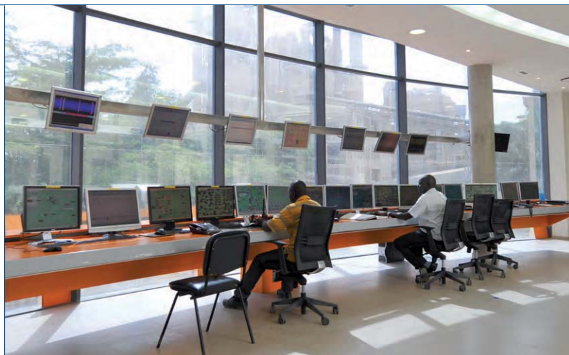
▲ Control room of the Sococim Industries cement plant in Rufisque.
