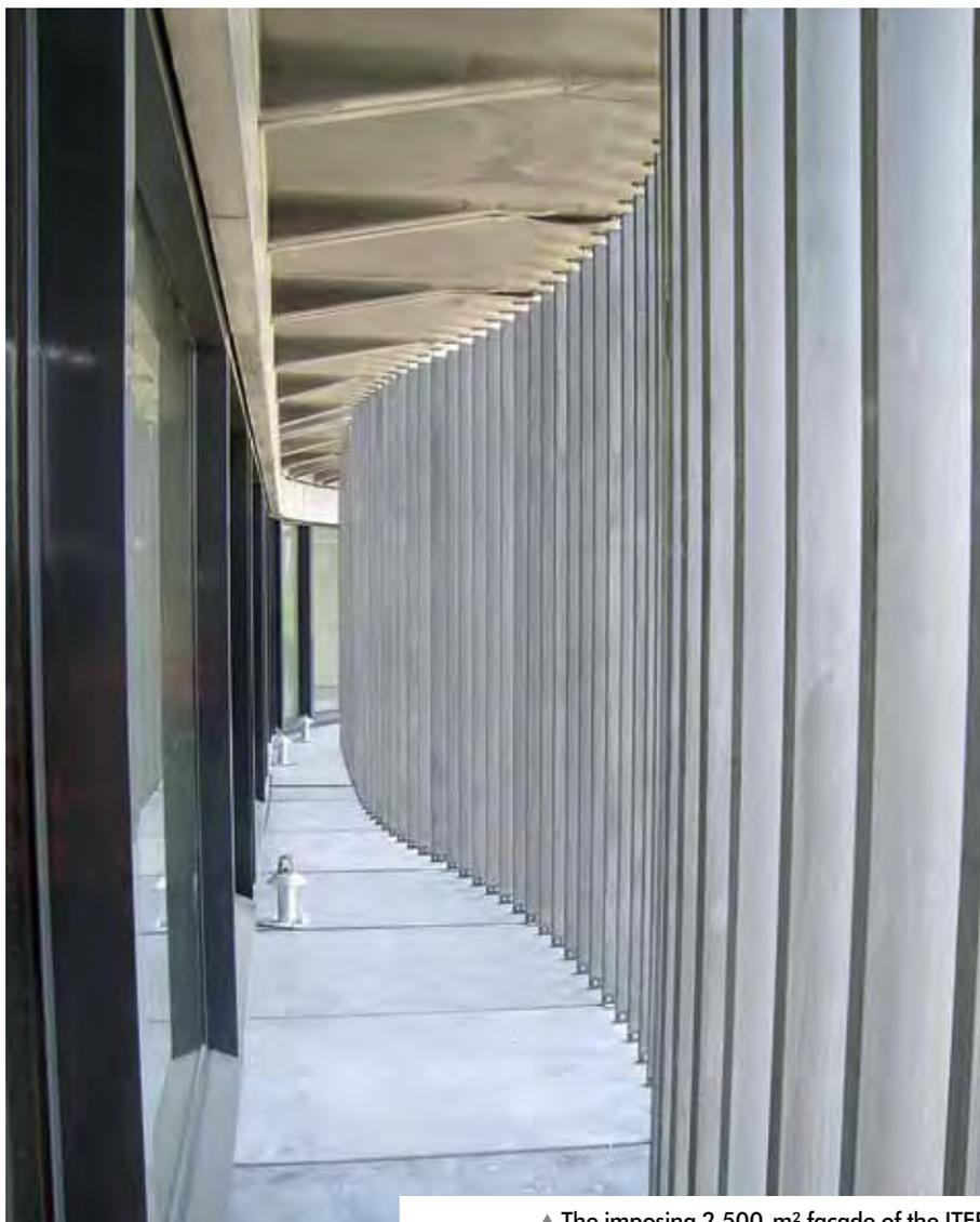
▲ The imposing 2,500-m<sup>2</sup> façade of the ITER administrative building at the Cadarache facility (France) consists of 2,000 high-performance concrete units in 100 different dimensions.
