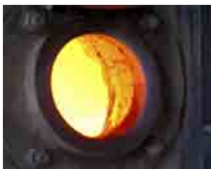
▲ Viewing port on a cement kiln.
