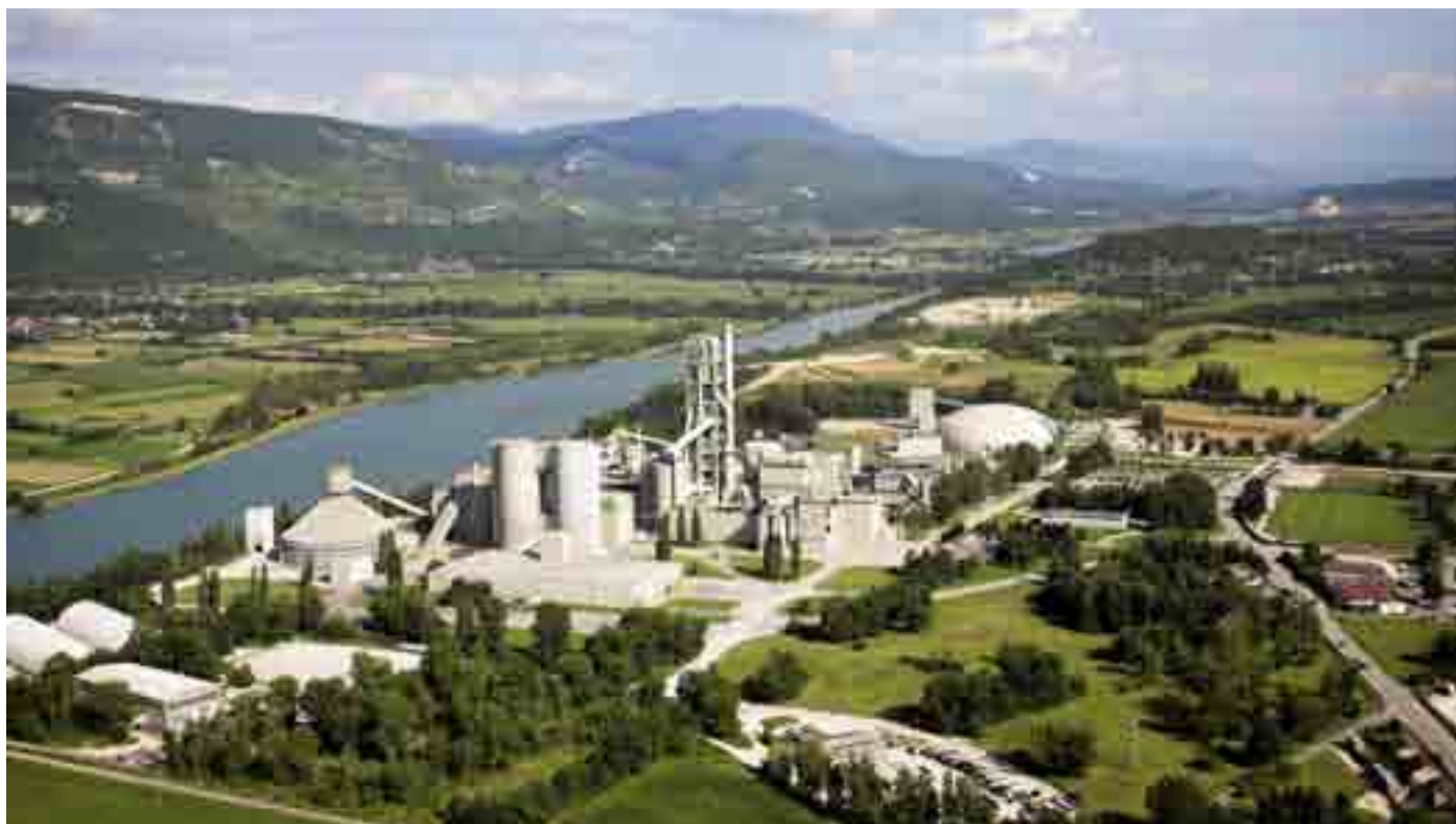
▼ The Montalieu cement plant in France's Alpine region.
