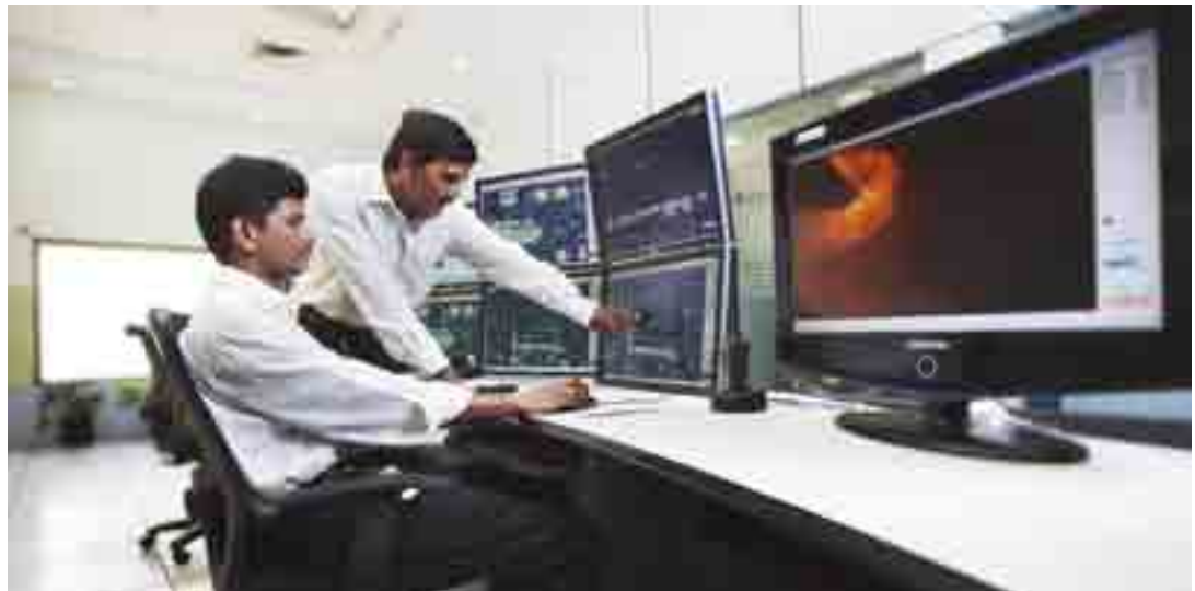
► Control room of the Bharathi Cement plant (India).
