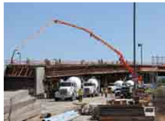
▲ Construction of a bridge over Lassen Street in Chatsworth.
