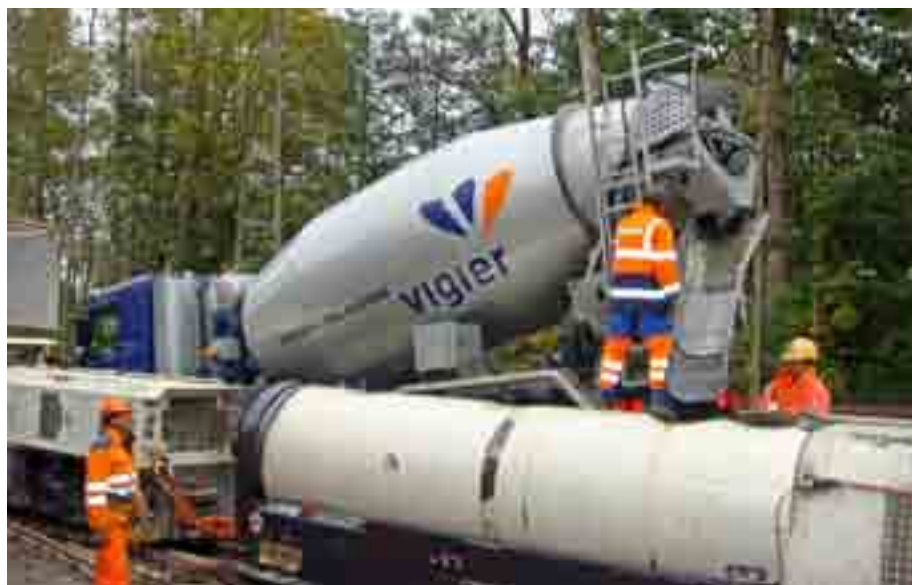
► Vigier Beton supplied concrete for a flood-relief tunnel.
