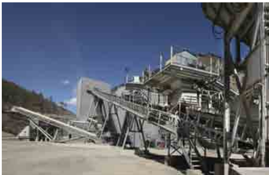
► Plant at the La Courbaisse: aggregate quarry in the hills above the French Riviera.
