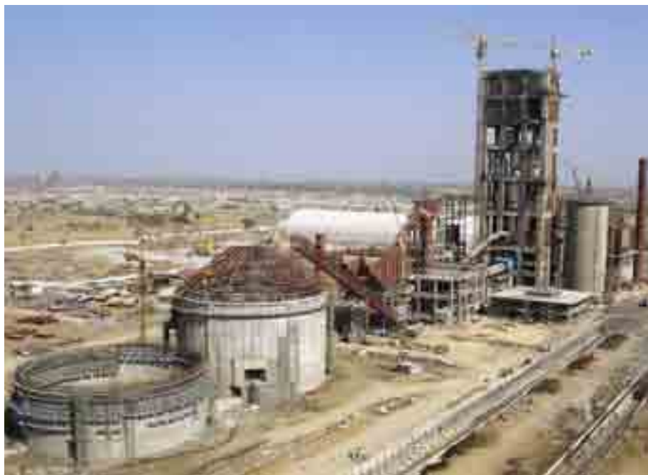
▼ Vicat Sagar Cement construction site in Karnataka, March 2012.
