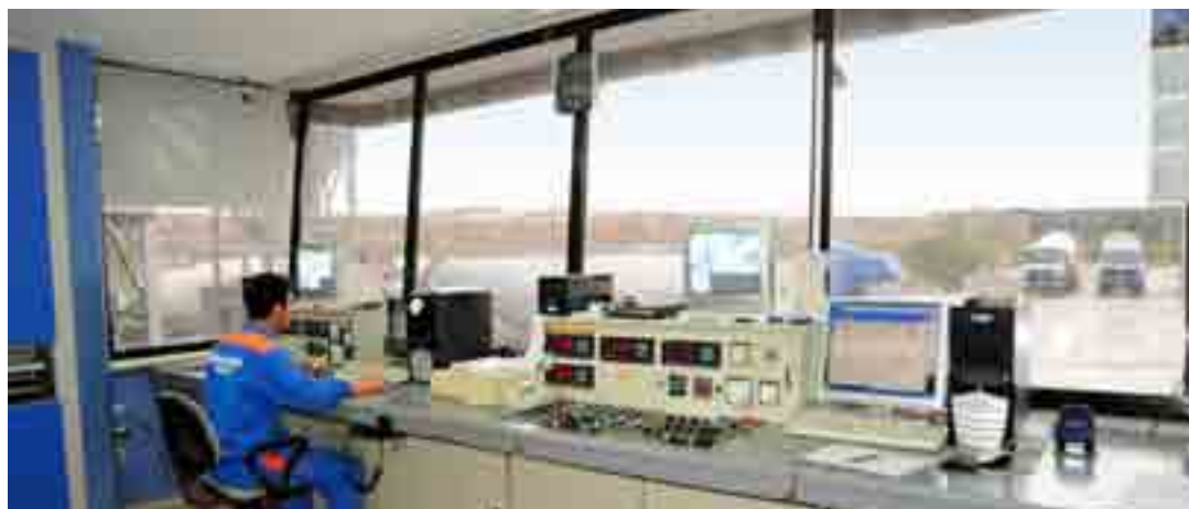
▼ Control room at the Merkez concrete batching plant (Turkey).
