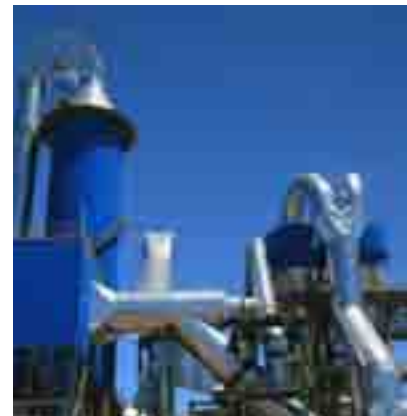
▲ Dedusting system on the raw meal crusher at the Jambyl Cement plant in Mynaral (Kazakhstan).
