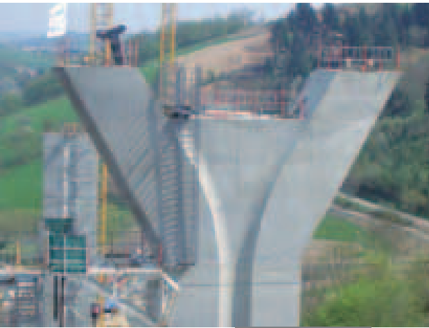
A89 motorway project, Lyons area.
