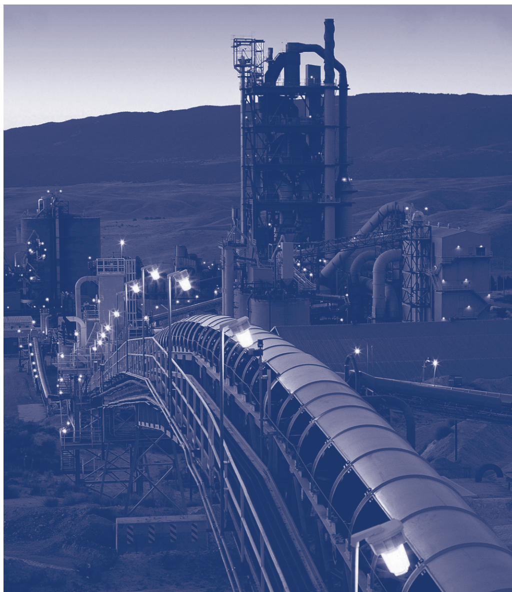
▲ Lebec cement plant in California (USA)
